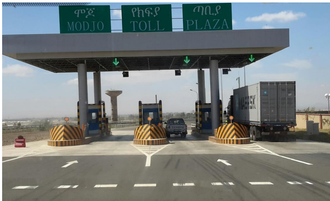
Toll Booth on new highway south of Addis Ababa December 2014.
